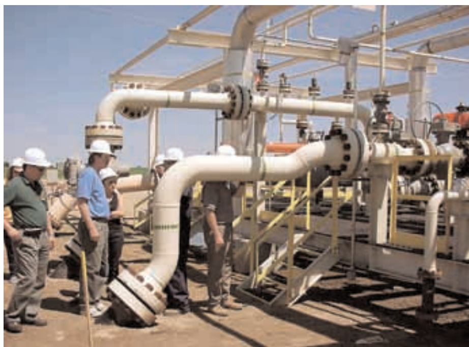
Ariba, Photo of point where CO 2 exits the underground pipeline that transports CO 2 from Beulah, ND to Weyburn, Saskatchewan. Courtesy of PTRC and the IEA GHG Weyburn CO 2 Monitoring and Storage Project
