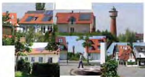
Several PV systems are connected to the low voltage grid
